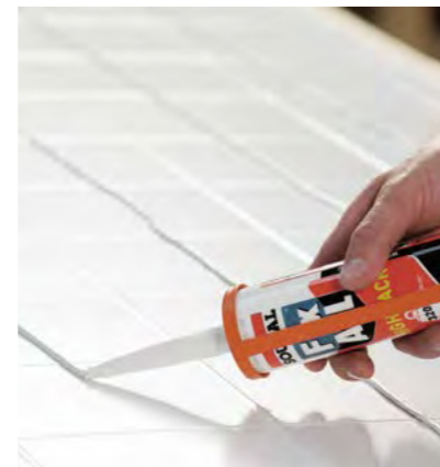
6. Apply adhesive to panel
