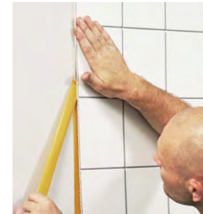
8. Once panel is in place remove the tape from behind the panel
