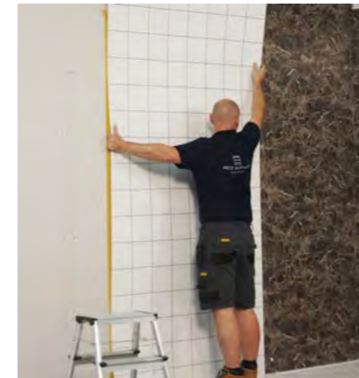
7. Fold top and bottom of tape over to reveal joint point then position panel
