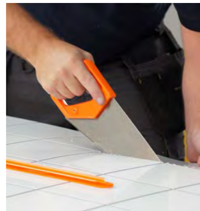
5. Trim panel using a knife or saw
