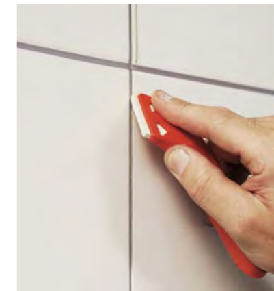
11. Wipe off excess sealant along the joint.
